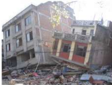
Collapse of RC frame buildings in Kathmandu
